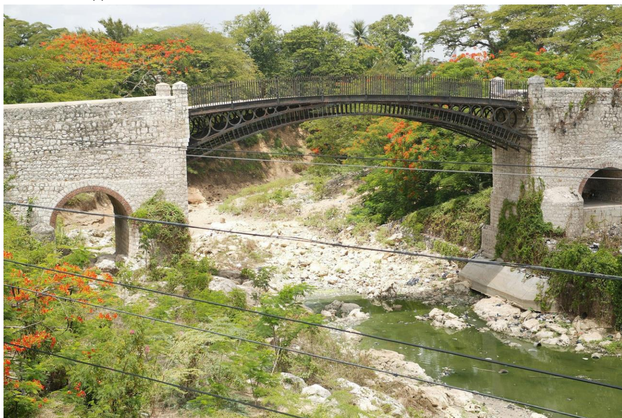
The Historic Cast Iron Bridge Across the Rio Cobre. Image courtesy of The National Library of Jamaica
