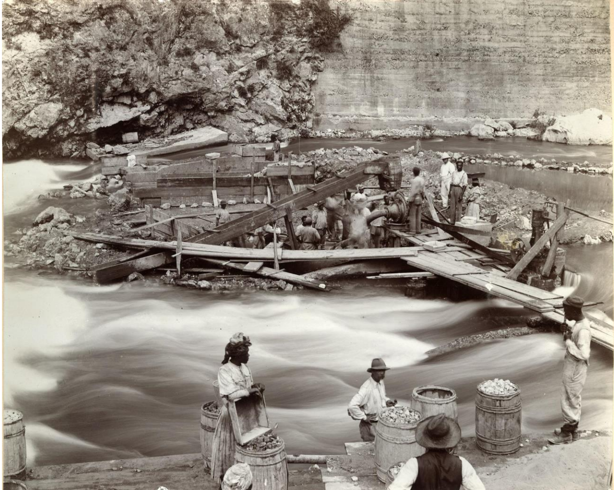
Early Work (1871-1876) on Building the Dam to Harness the Water of the Rio Cobre. Image courtesy of The National Library of Jamaica
