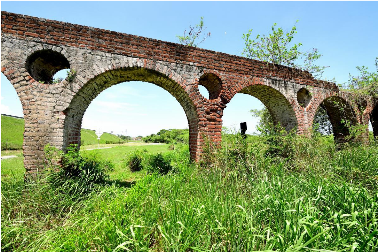
The Bushy Park Aqueduct which Channeled Water from the Spring Garden River to Power the Water Wheel at the Sugar Factory. Image courtesy of JNFoundation
